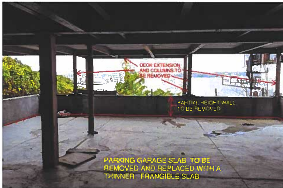
Figure 2 - Slab Removal & Replacement
